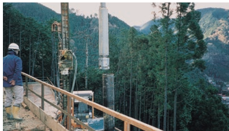
Piling After casing through the collapsing overburden, insert a H-steel, then pull up the casing.
